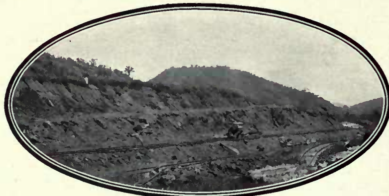
Where the two men are standing was the bottom level in Culebra Cut which the French company reached. The motor car is on a level sixty-five feet lower which represents the digging done by the United States in this section of Culebra Cut.
