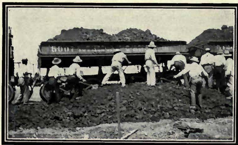
Dumping a Car Load of Spoil.
