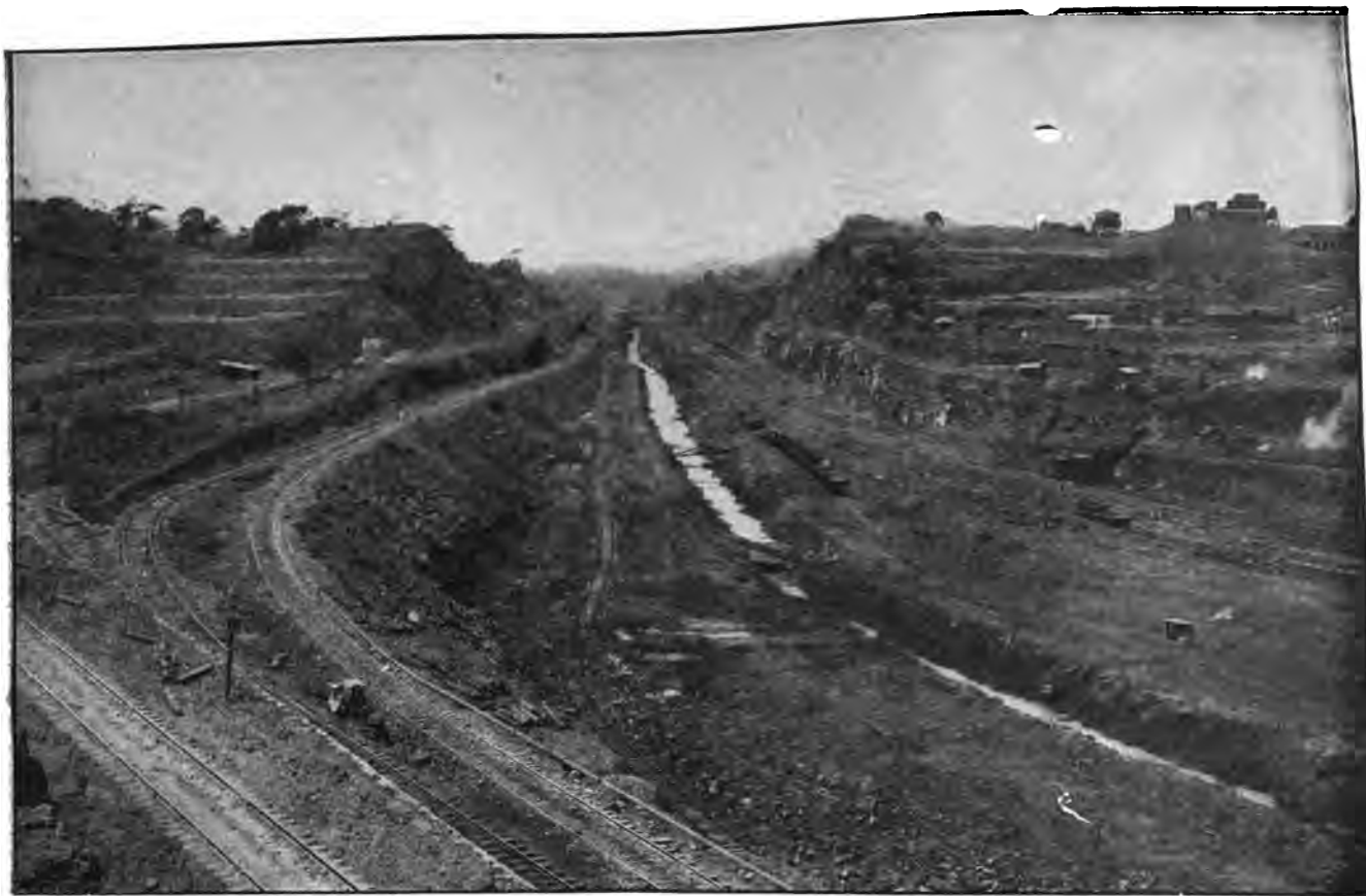
CULEBRA CUT LOOKING NORTH FROM CUNETTE.
