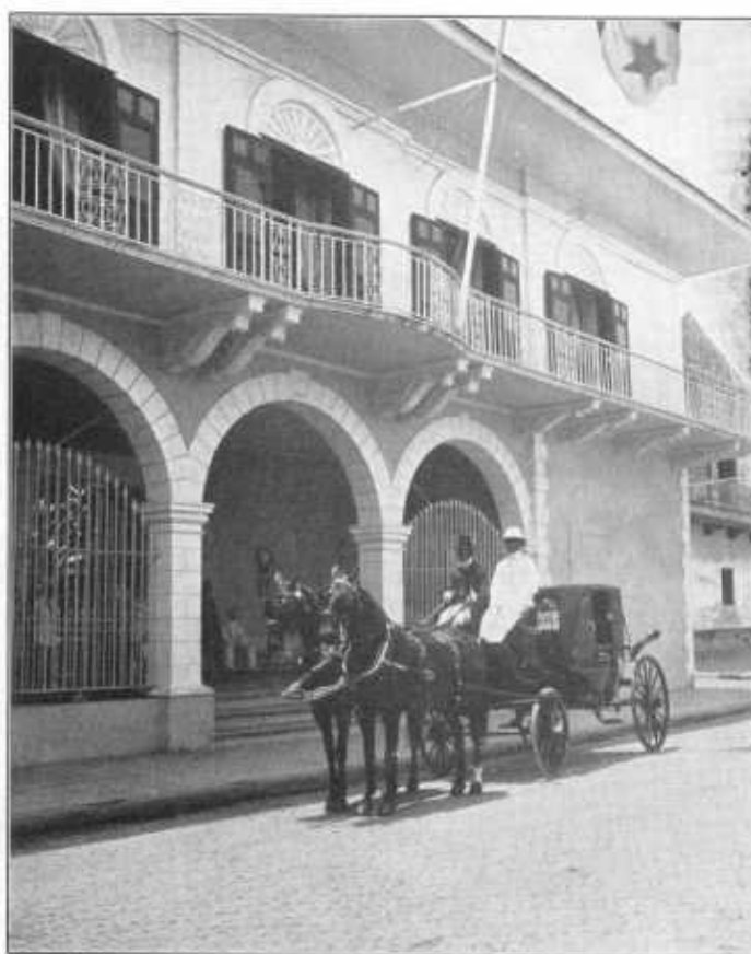
Residencia Presidencial (Exterior) Presidential Residence (Exterior View)
