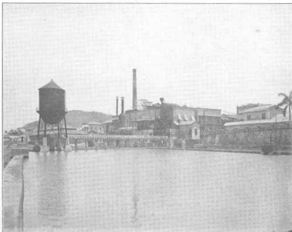
Vista General de la Planta.—Panama-American Corporation General View.—Panama-American Corporation Plant
