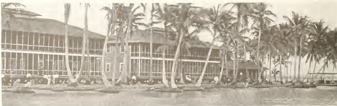
Bachelor Quarters at Toro Point (Pre 1913)
