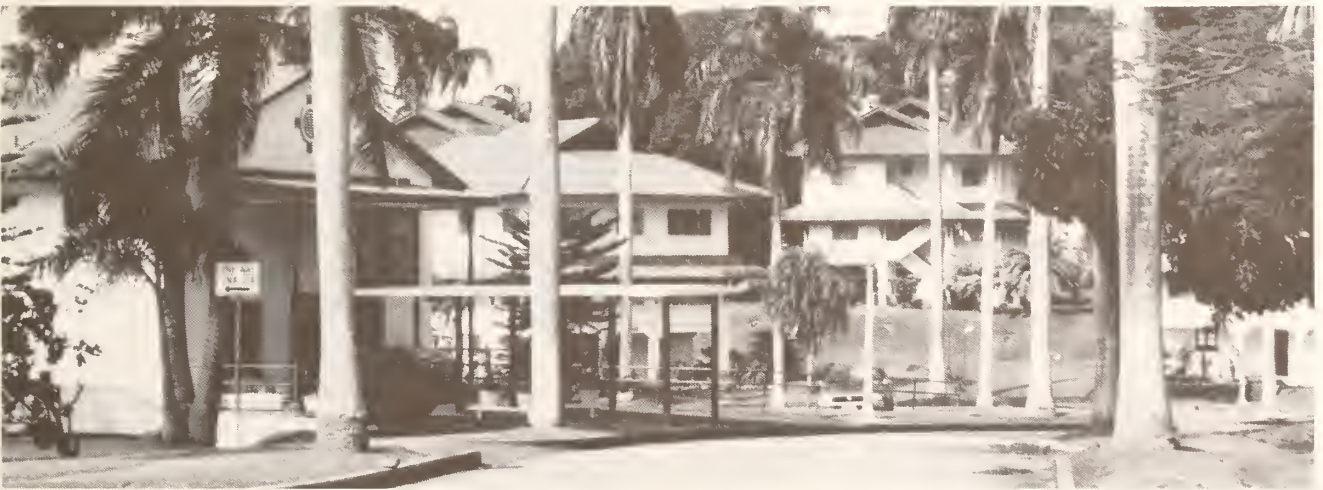
View down residential street, Albrook Field, C.Z.
