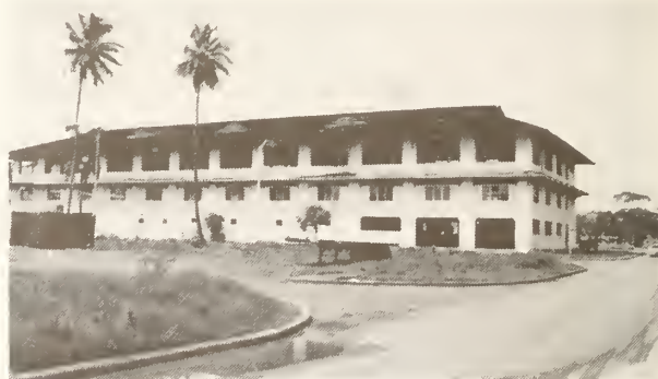
Former Administration Building
