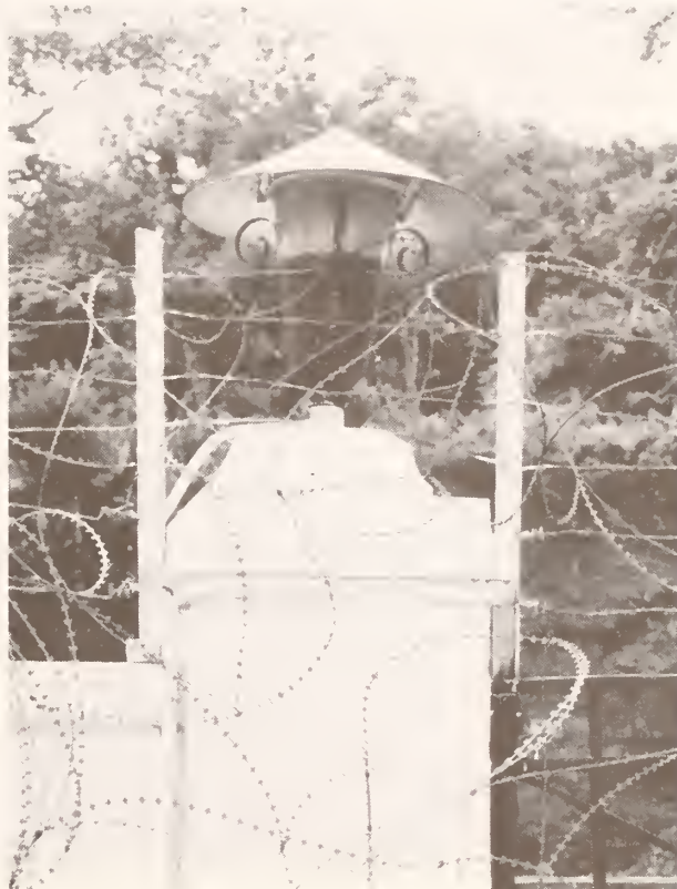
Entry light/gate detail
