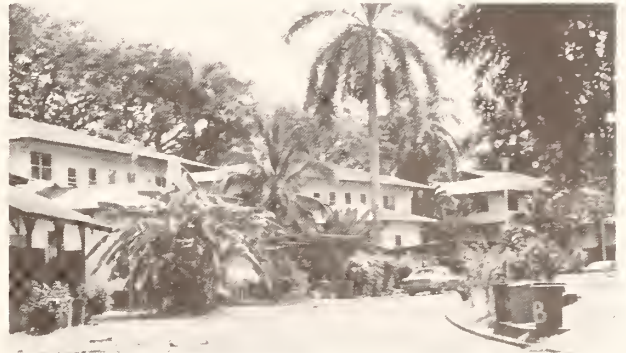
Residential quarters at Fort Clayton
