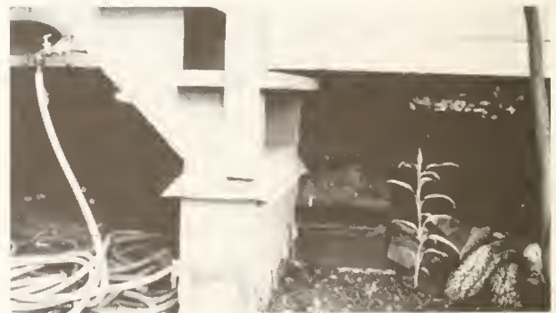
Raised structure with metal flashing serving as termite shield
