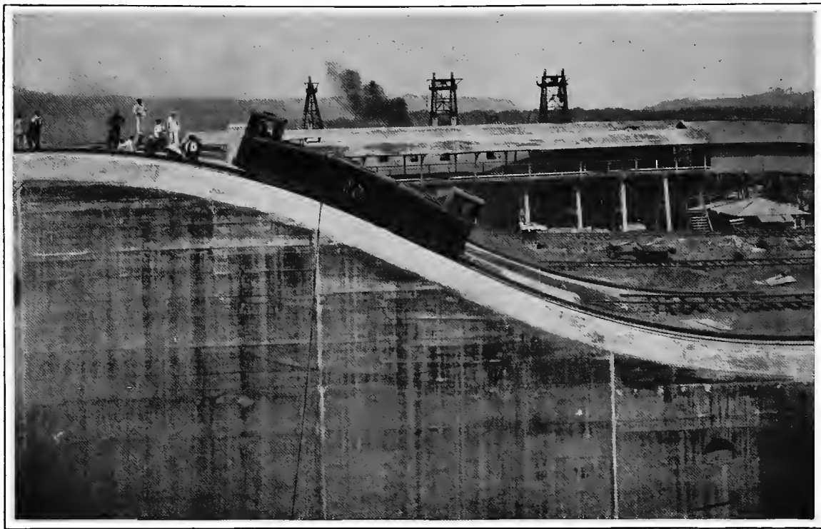
AN ELECTRIC TOWING LOCOMOTIVE IN ACTION
