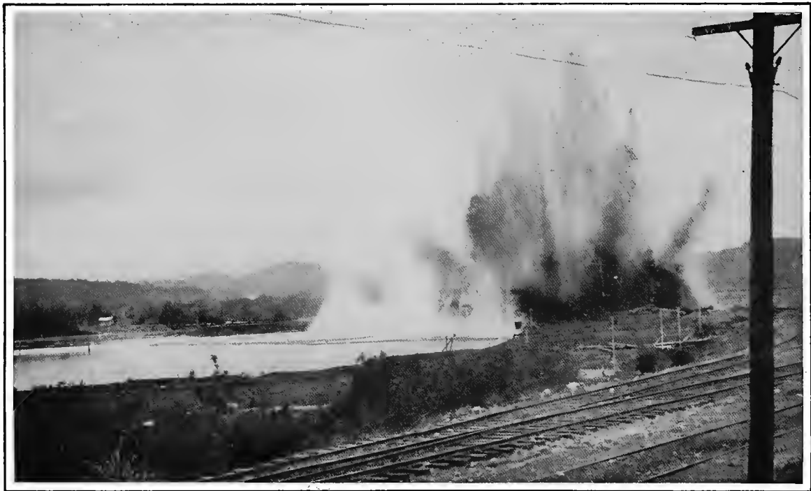
BLOWING UP THE SECOND DIKE SOUTH OF MIRAFLORES LOCKS
