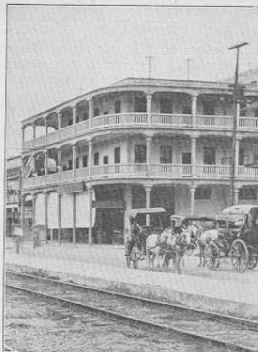
One of the newer type of concrete buildings. This structure is the property of the Panama Railroad, which owns most of the land in Colon.
