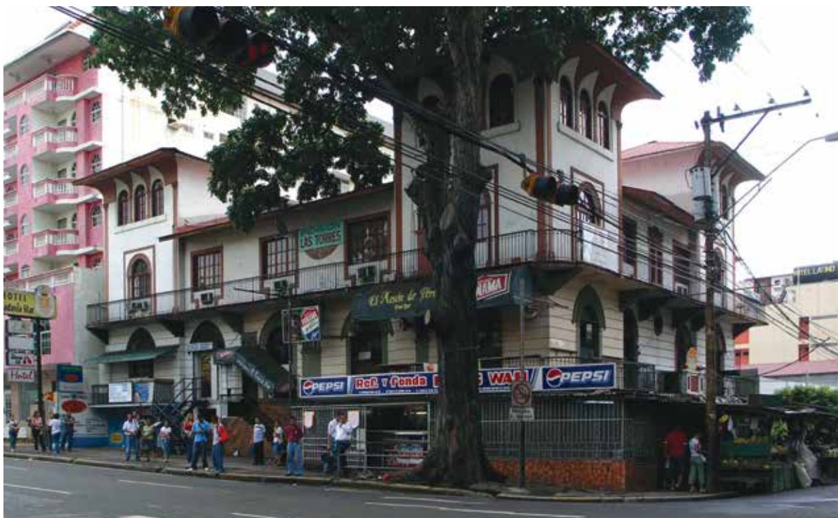
Fig. 61 La antigua residencia de Guillermo Patterson, ubicada en avenida Perú y calle 36 Este, y construida en la década de 1930, es el ejemplo más significativo en Panamá del palacete neohispánico de torres esquineras con miradores. Hoy, sus virtudes arquitectónicas son difíciles de apreciar por los incontables añadidos y letreros, pero sería fácilmente recuperable. | The former residence of Guillermo Patterson, located on Peru Avenue and 36 East Street, and built in the 1930s, is the most significant example in Panama of the Neo-Hispanic palace of corner towers with viewpoints. Today, its architectural virtues are difficult to appreciate by the countless additions and signs, but they could be easily recovered.
