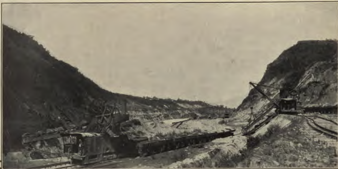
CULEBRA CUT IN 1904, DECEMBER, LOOKING NORTH. FRENCH EQUIPMENT USED BY WALLACE.
