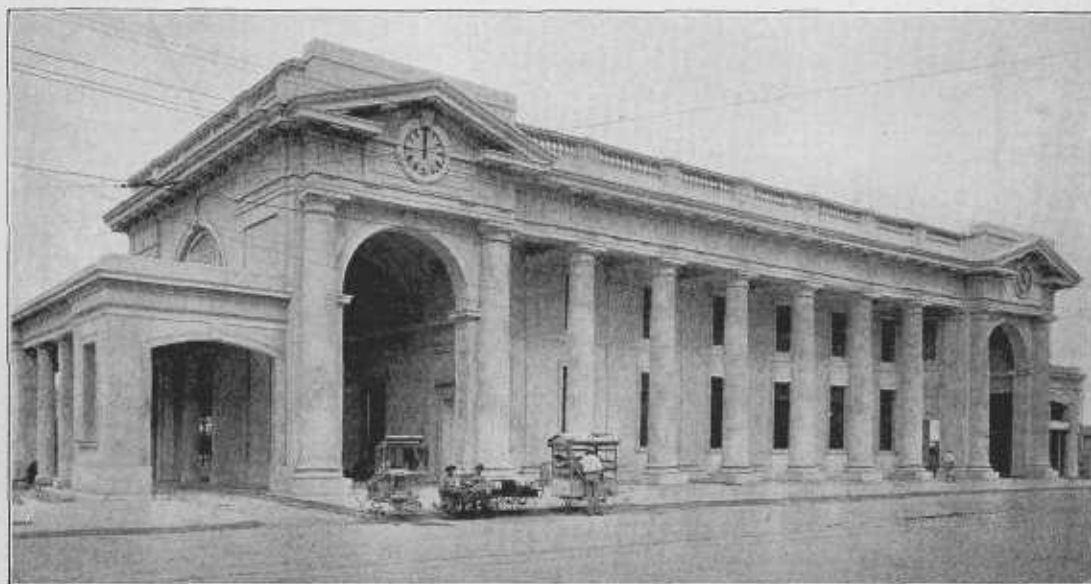
New Panama railroad passenger terminal in Panama, just completed.
