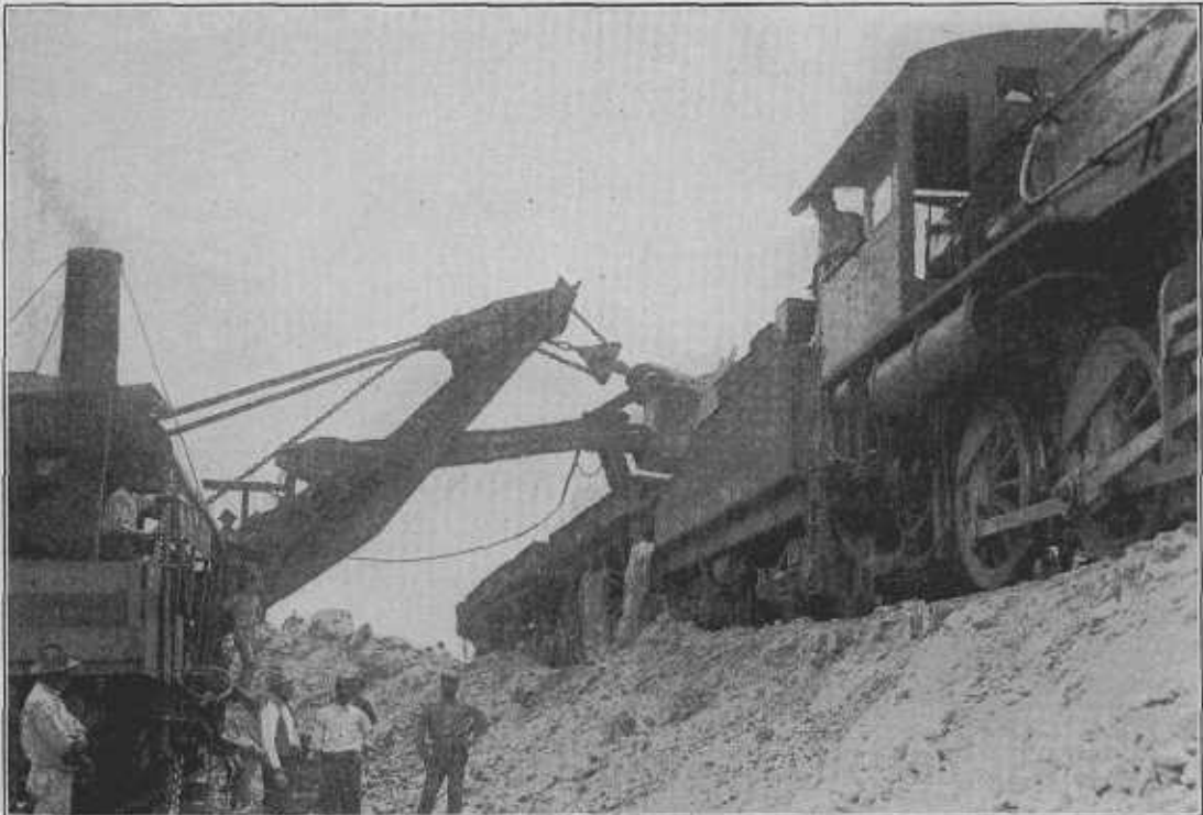
Loading dirt train for trestle fill.
