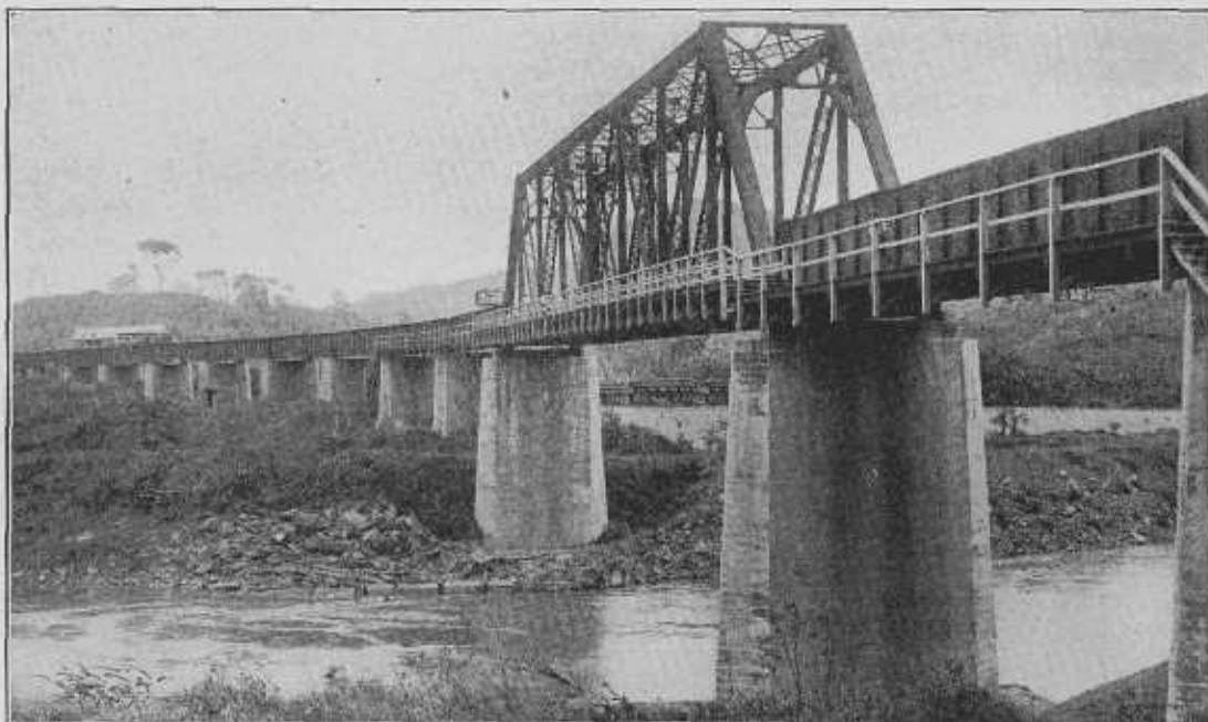
The largest railroad bridge on the new line, spanning the Chagres River at Gamboa. It is 1,320 feet long. The Chagres River empties into the Canal at this point.
