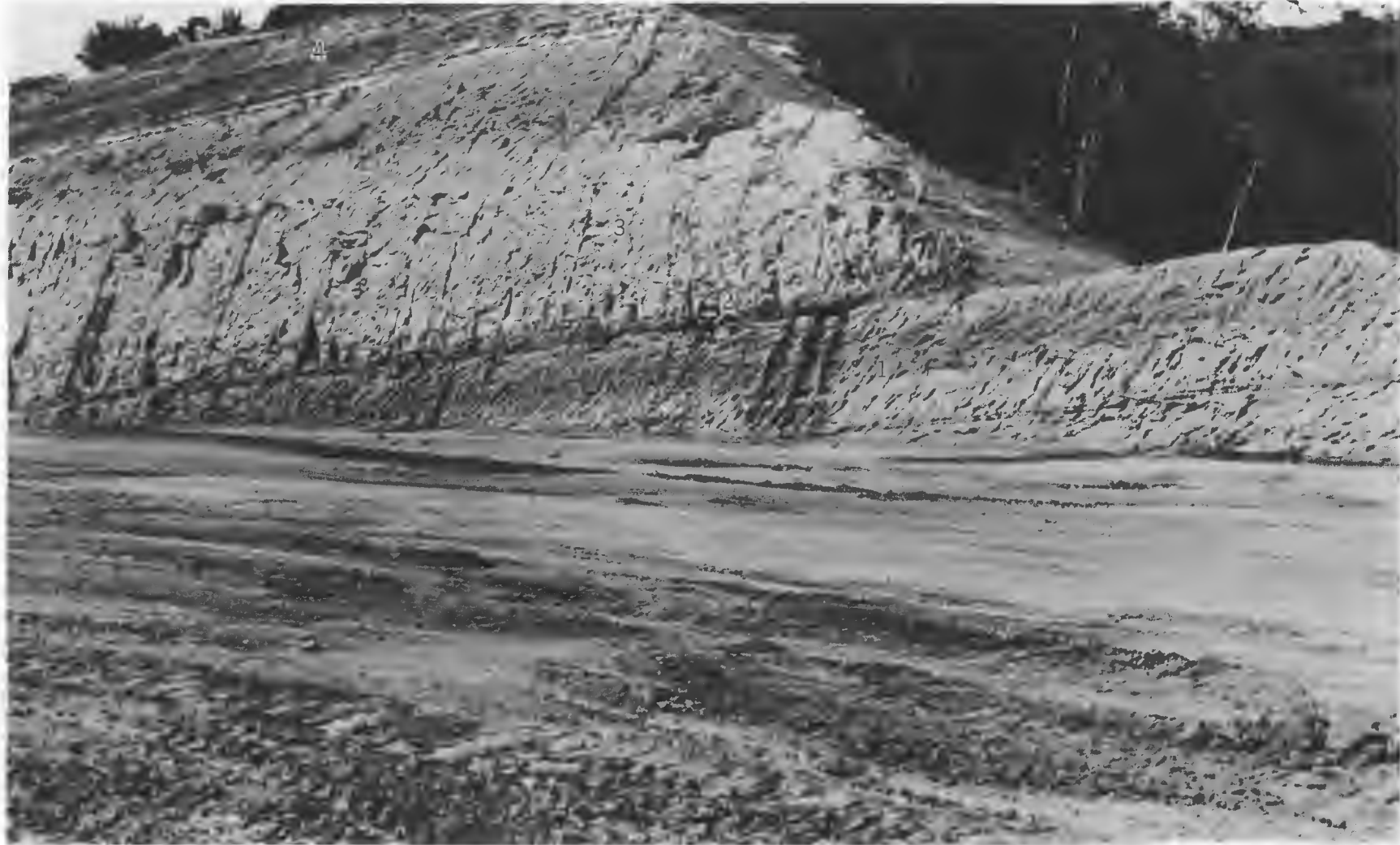
STRATA IN MIDDLE PART OF GATUN FORMATION ON EAST SIDE OF GATUN THIRD LOCKS EXCAVATION, CANAL ZONE The numbered units correspond to those of the stratigraphic section. Photograph by Geological Section, Special Engineering Division, Panama Canal Company.
